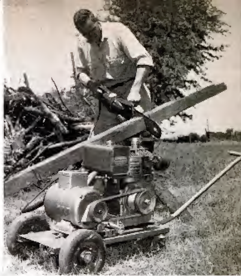
Electricity from the generator drives an electric saw
